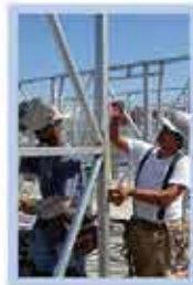
Metal decking w/concrete
